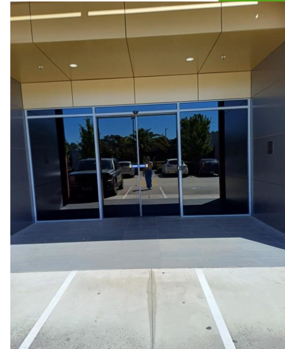
Right Image: The accessible entrance at the back of the building. This entrance has no stairs.
