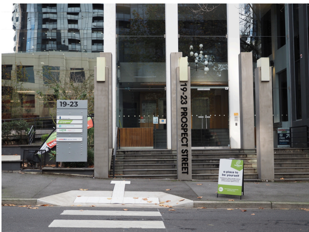
Image Description: Exterior of 19-23 Prospect St, in which headspace Box Hill is located on level 1
