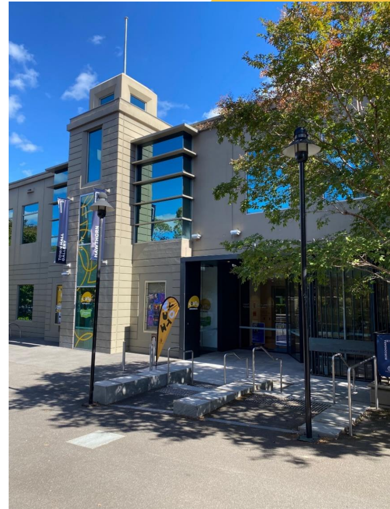
Image description: The building entry for headspace Hawthorn and the Hawthorn Arts Centre. Enter the glass door on the left to get to headspace Hawthorn on level 1. There are green signs for headspace Hawthorn and yellow signs for Boroondara Youth.
